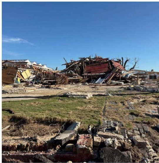
Left: Waterloo Great House, before and after Hurricane Melissa
