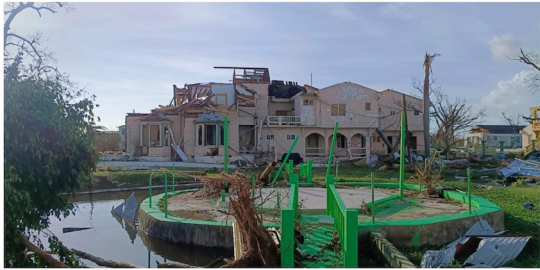
Left: Invercauld, before and after Hurricane Melissa
